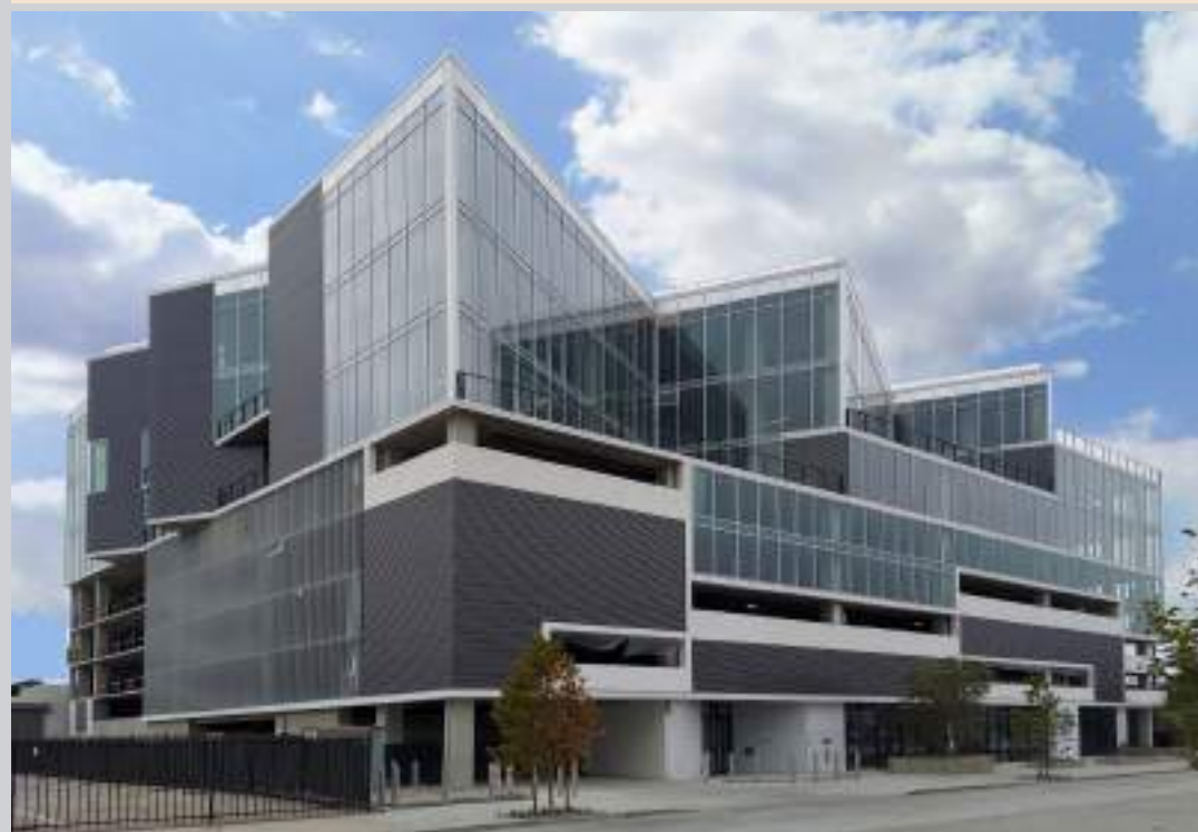
CW-700 Curtainwall with Solarban IG Units
