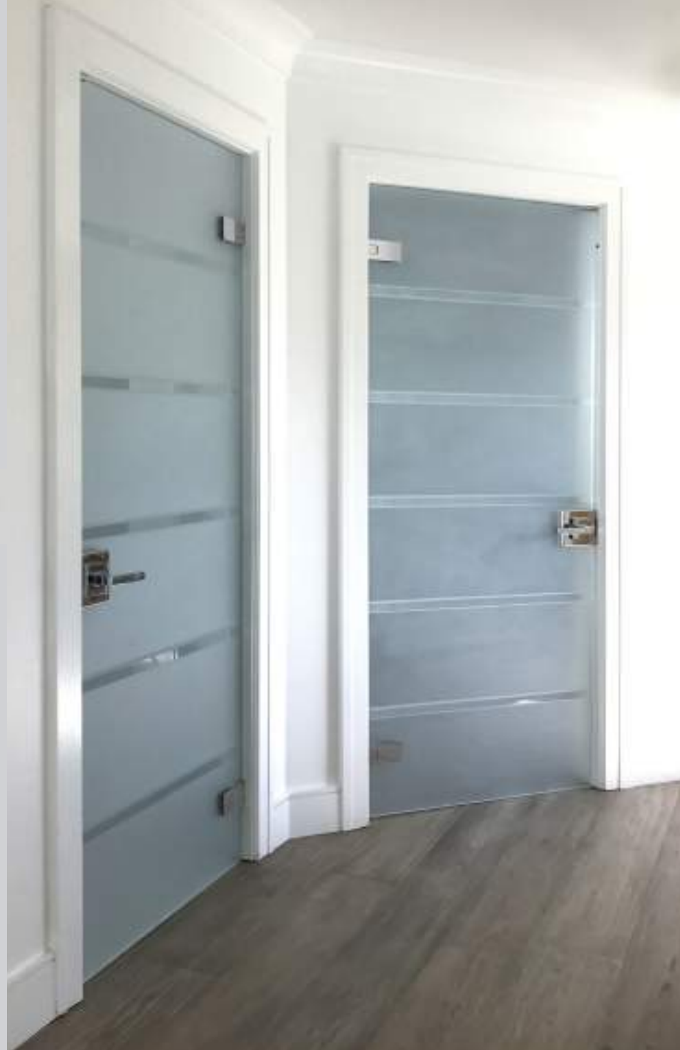
Interior Doors with Custom Sandblast Glass, Samson Hinge & Covina Housing Lock
