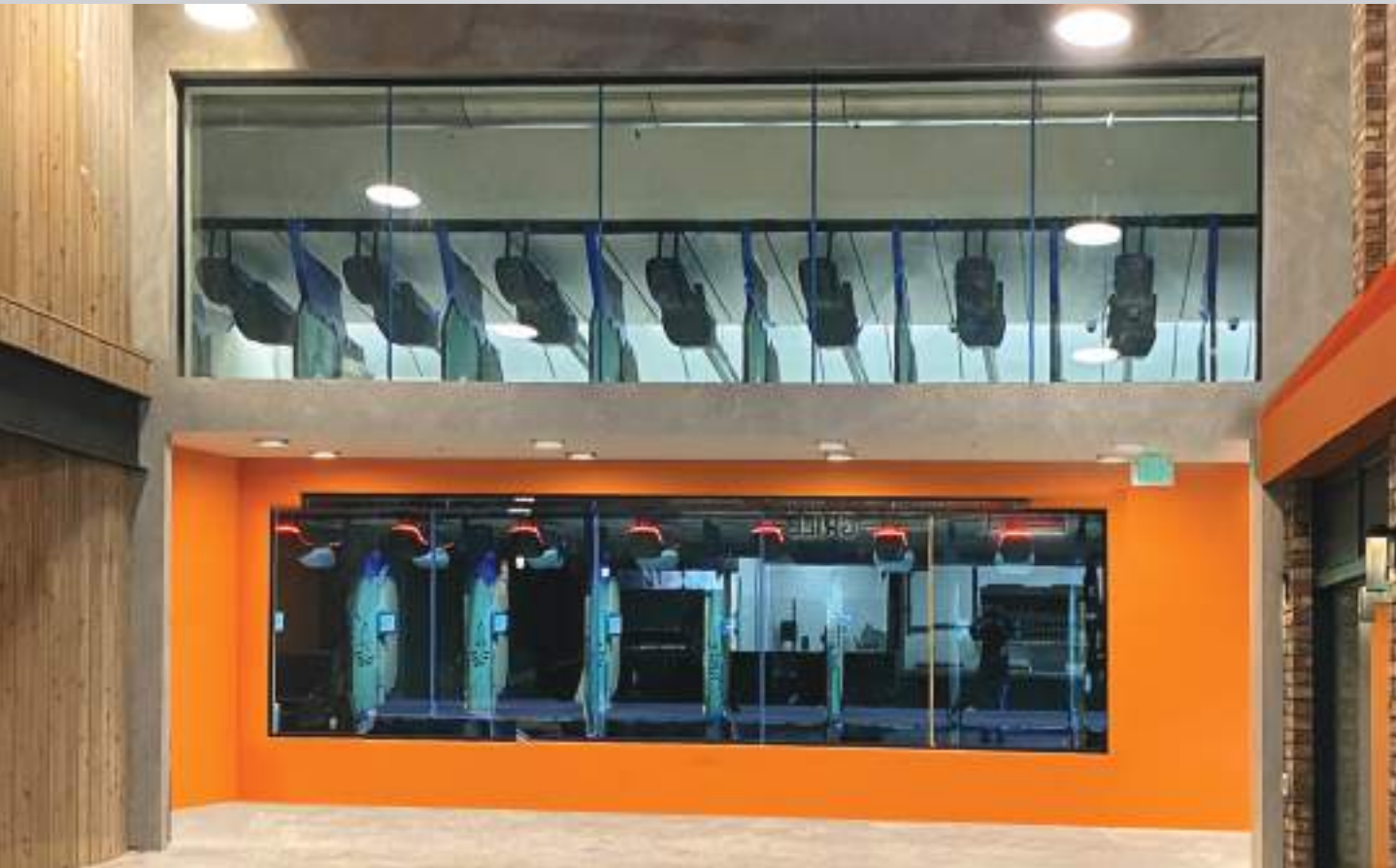
Fixed Glass Panels with Level 2 Bullet Resistant Glass
