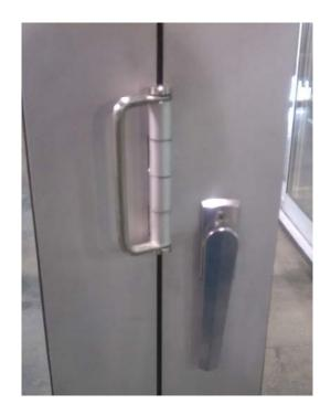
To operate folding leaves: Shown is the lock handle and pull handle (left side). The lock handle is shown in the locked position.
