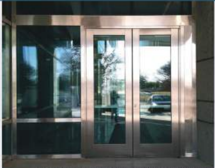
Full Frame Doors & Storefront Framing Cladded in Stainless Steel
