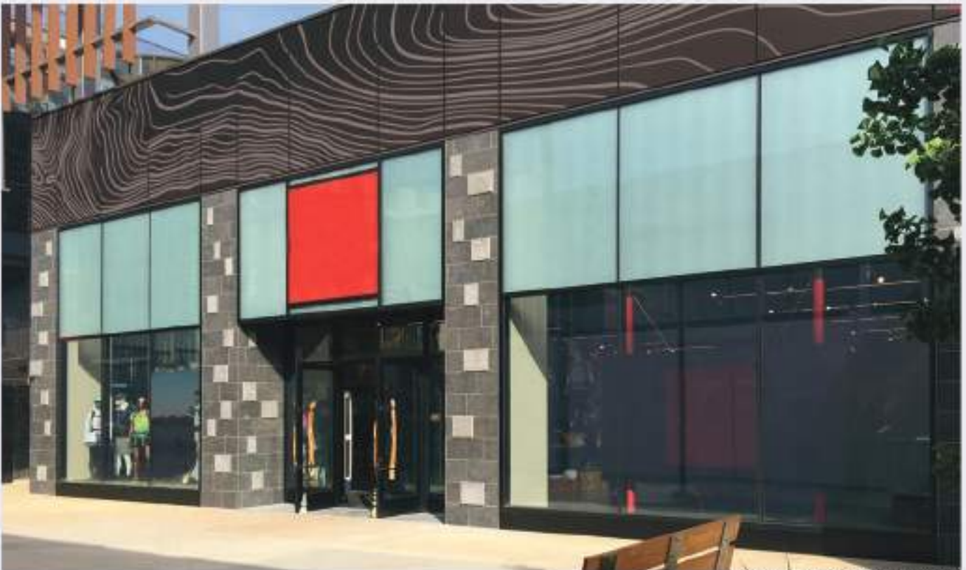
Storefront with Spandrel Infill Panels
