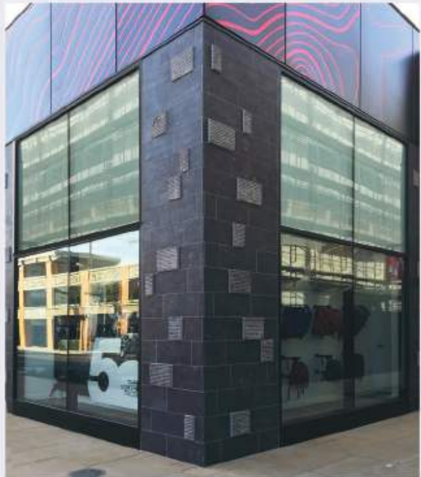
Aluminum Storefront with Insulating Low-E Glass Unit
