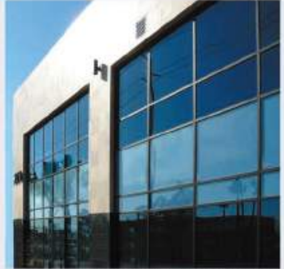
Curtainwall with Tinted & Spandrel Glass
