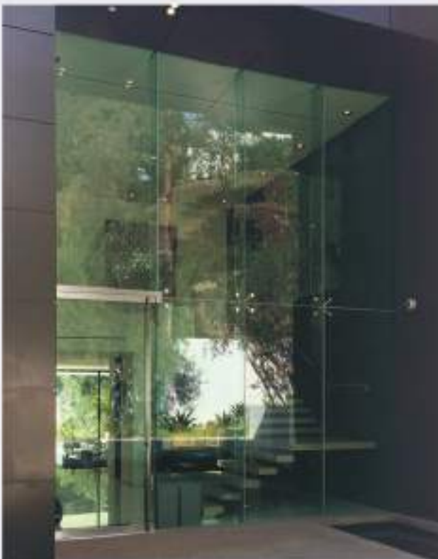
Glass Wall System with 3/4 Clear Tempered Glass
