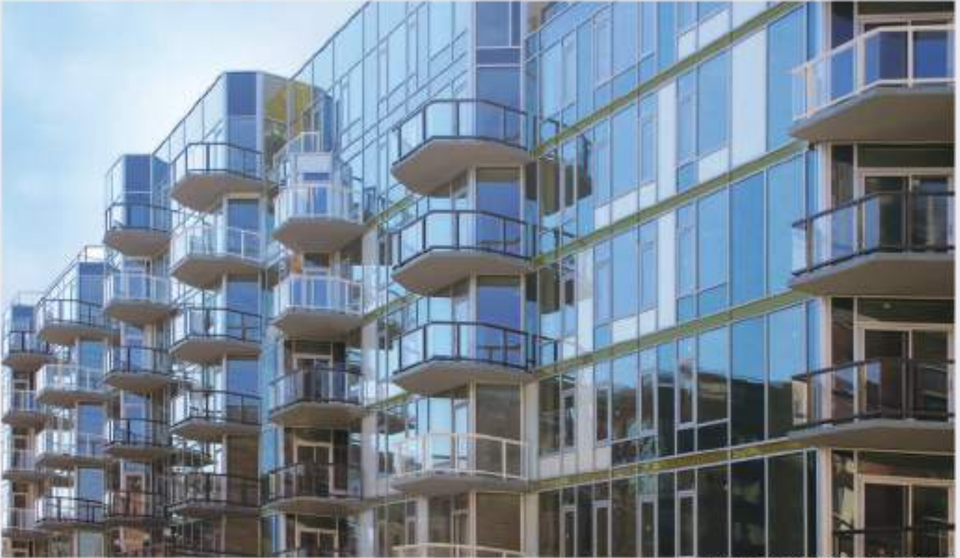
Curtainwall with Color Spandrel IG Units
