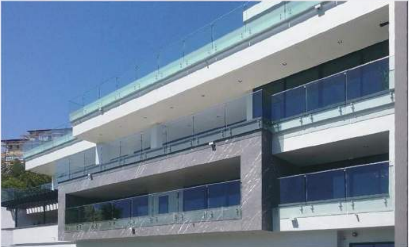
Handrail System with Tempered Laminated SentryGlas®
