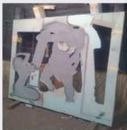
Custom Cut Glass Before Installation
