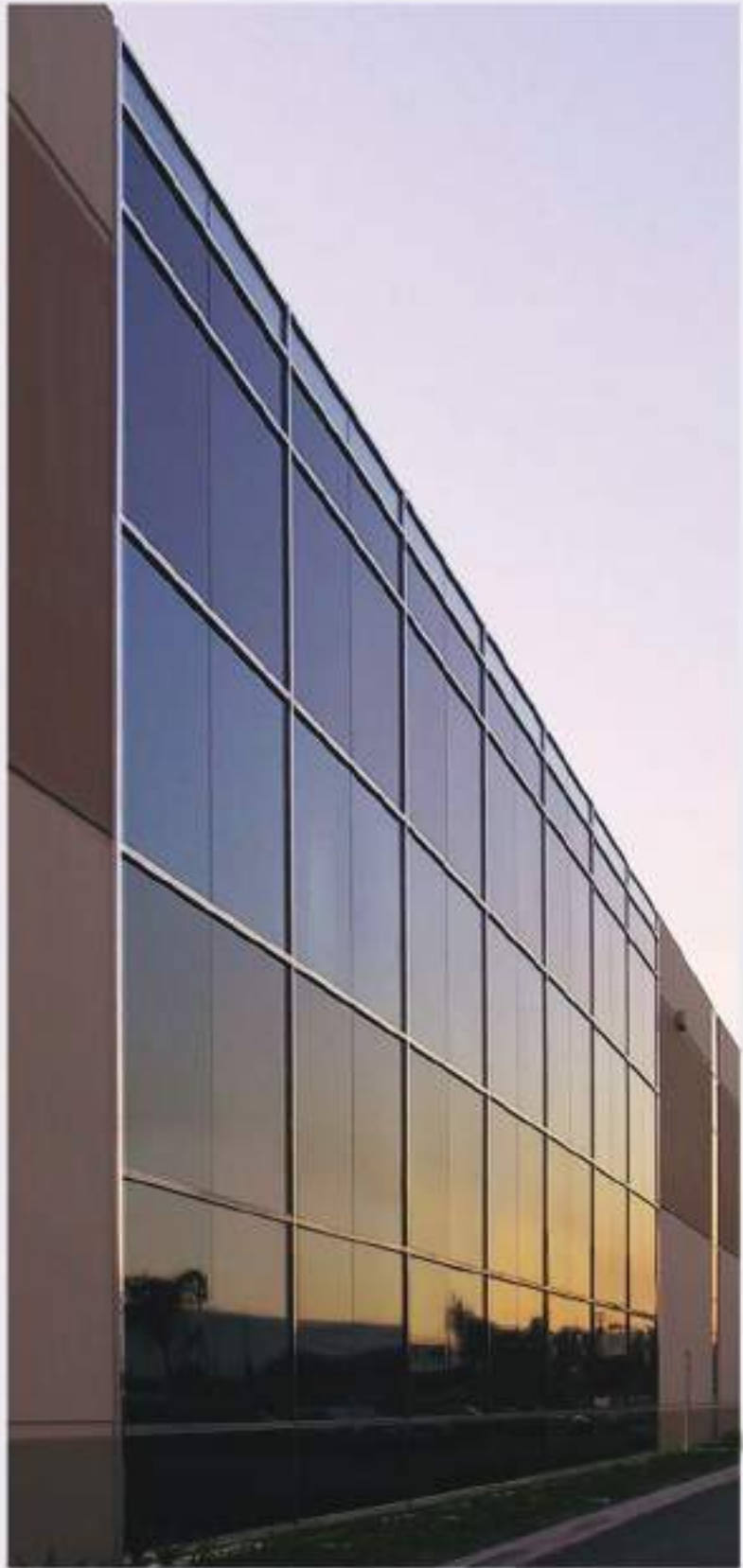
Aluminum Curtainwall with Reflective Glass IG Units
