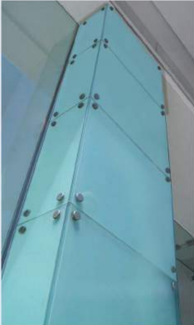
Spandrel Glass Panel Column Cover
