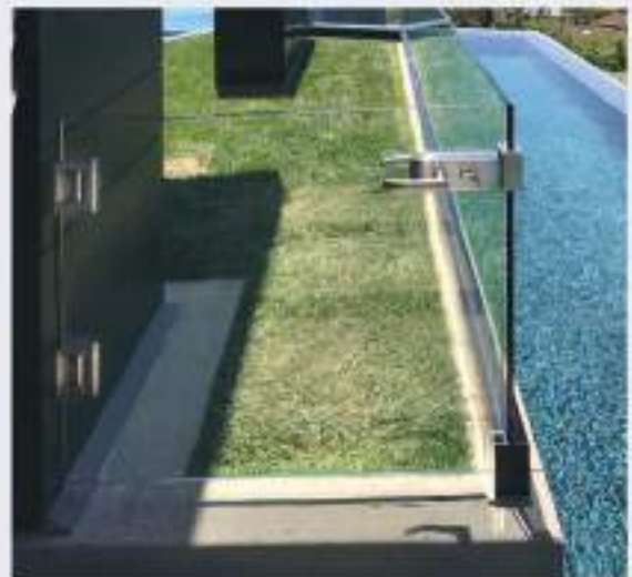
Security Gate with Custom Strike Application
